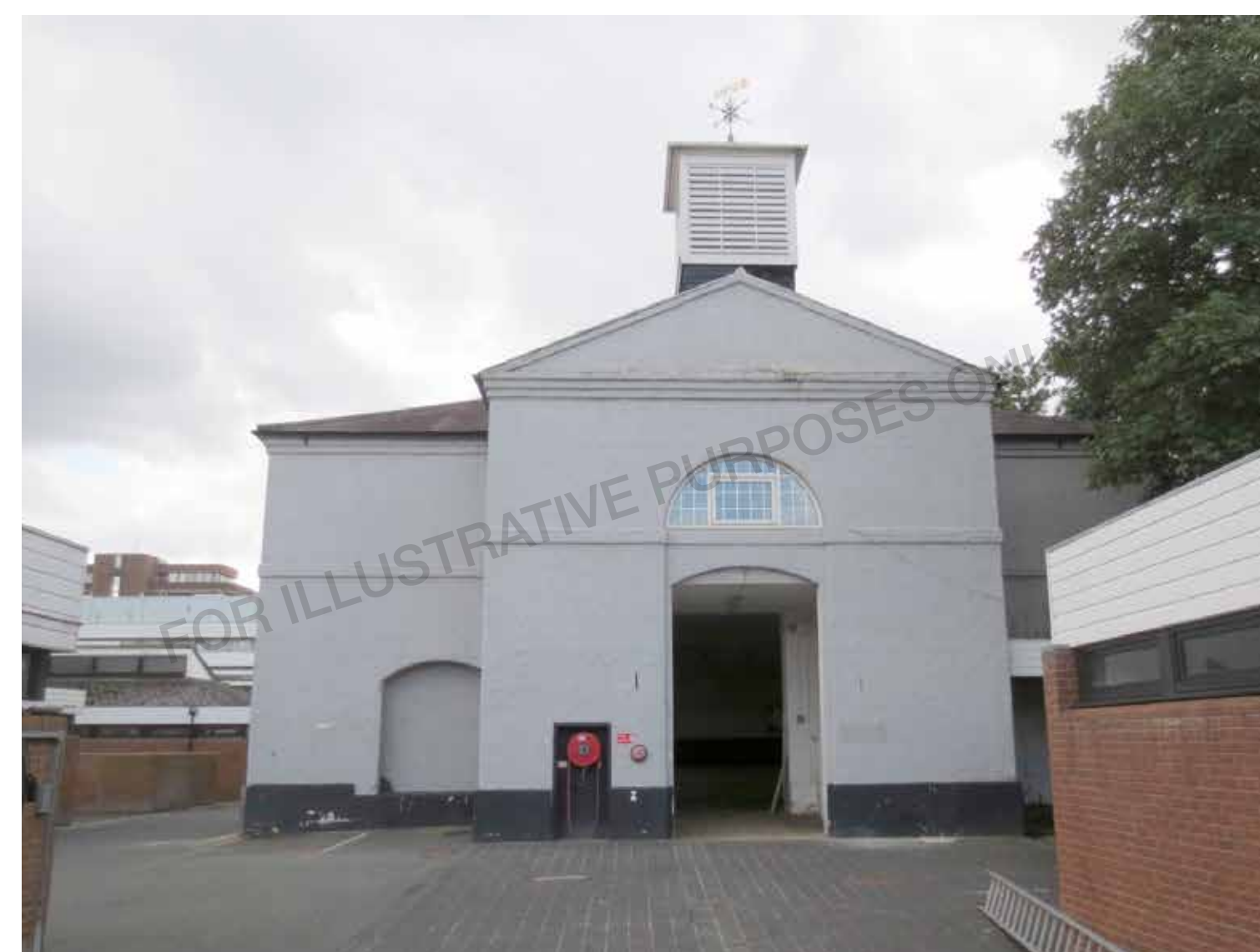
Existing pebble dash rendered elevation
