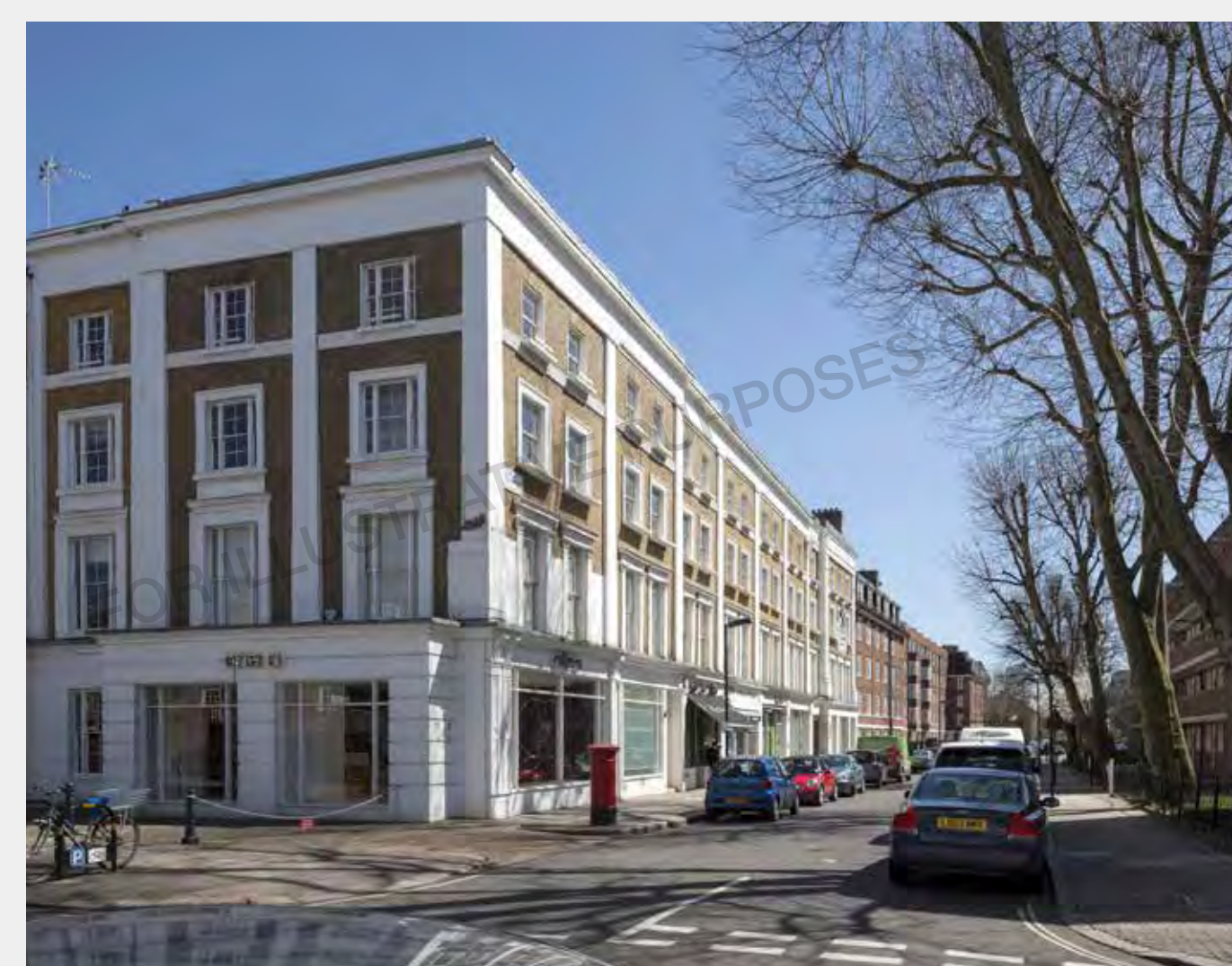
Existing view of Queen's Terrace
