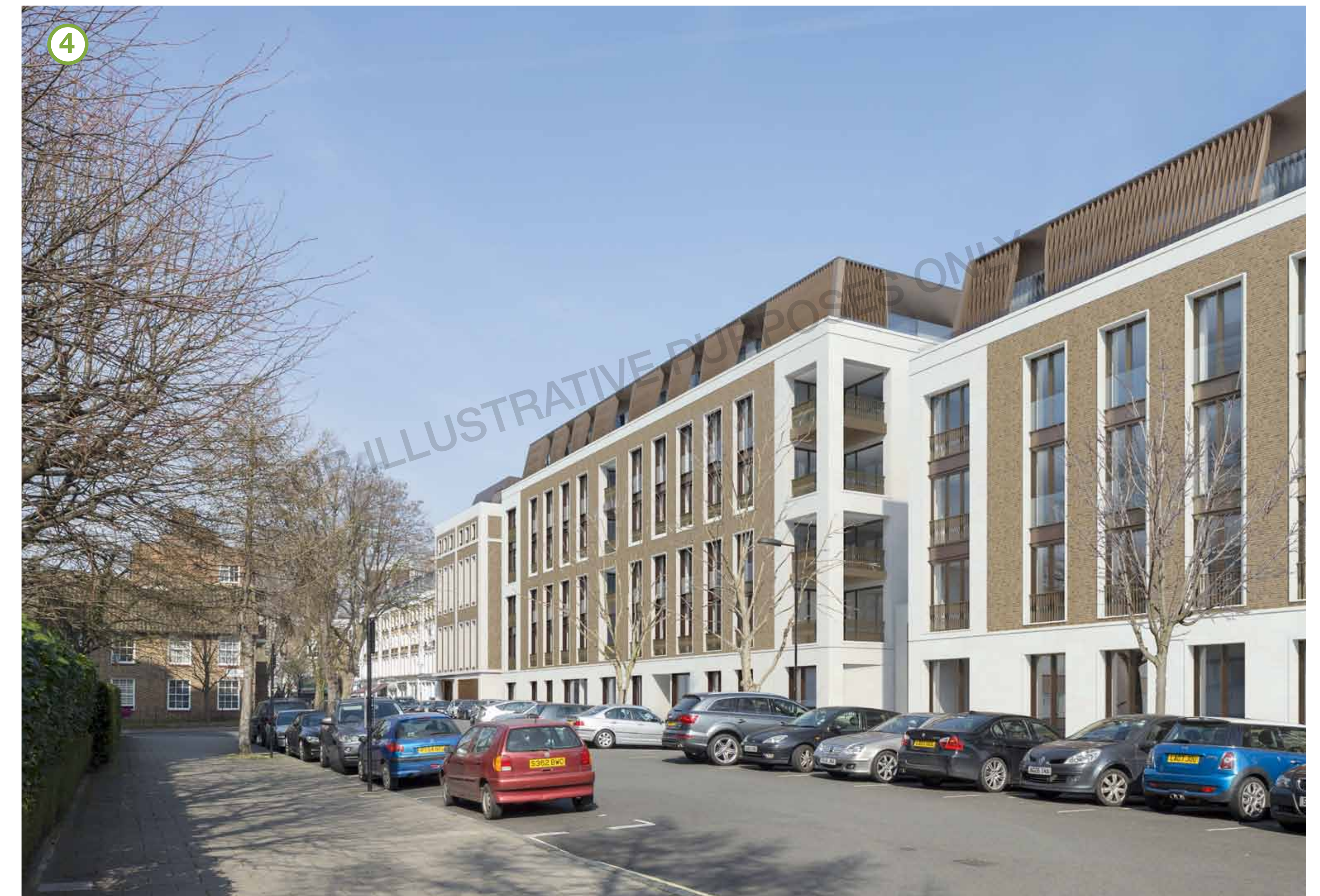
View 4 - Proposed view of Queen's Terrace (proposed improvements to Queen's Terrace omitted)
