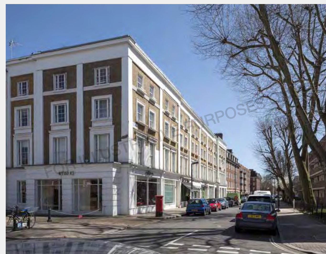
Existing view of Queen's Terrace
