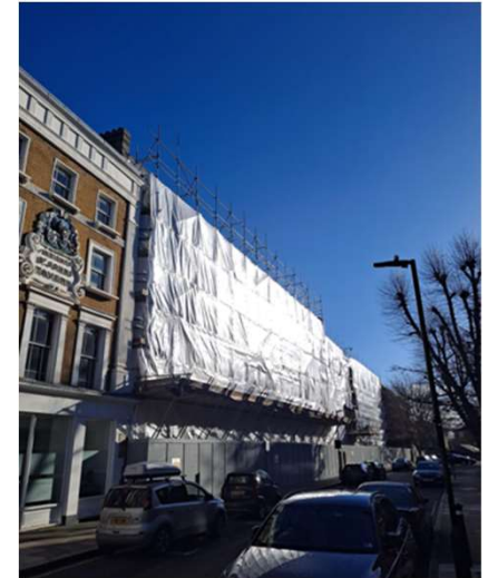
Jubilee buildings covered with scaffolding and screen
