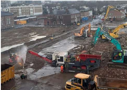
Sandvik crusher (red machine) breaking down material
