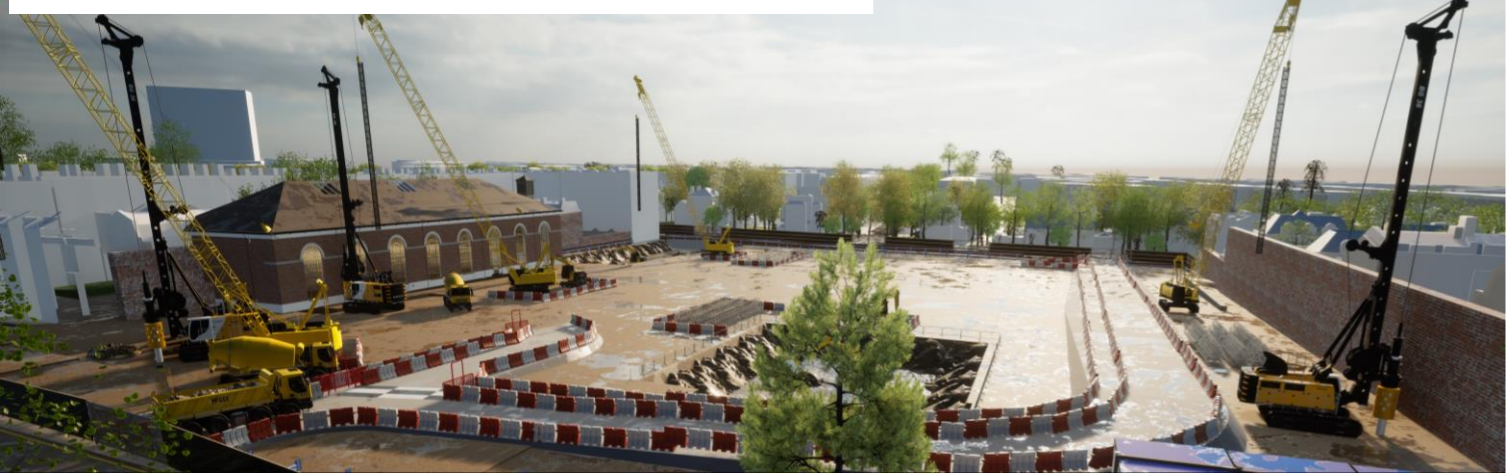
Computer generated image showing site with piling rigs in operation
